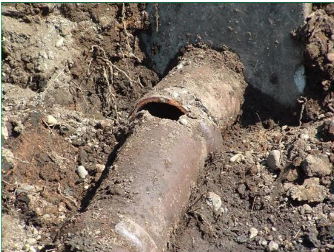
Damaged vitrified clay pipe sewer line.
