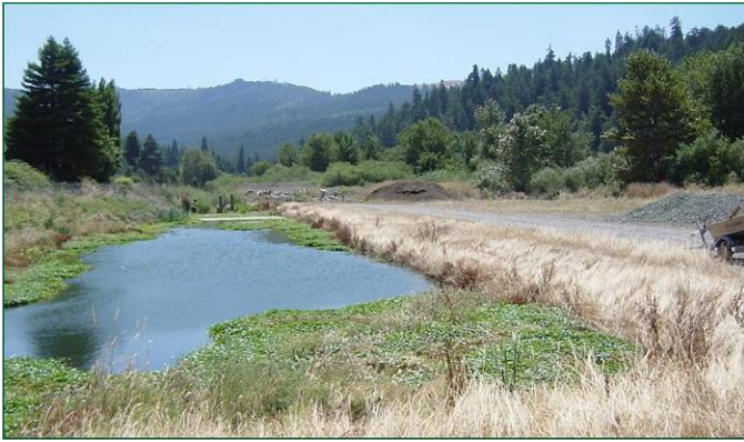
Scotia wastewater treatment pond.
