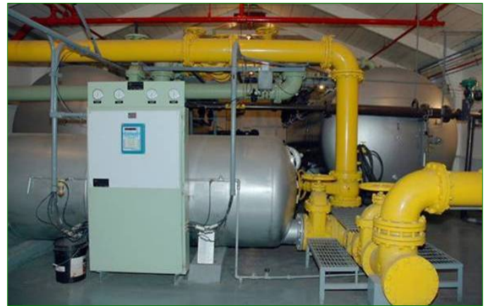
Scotia water treatment facility.
