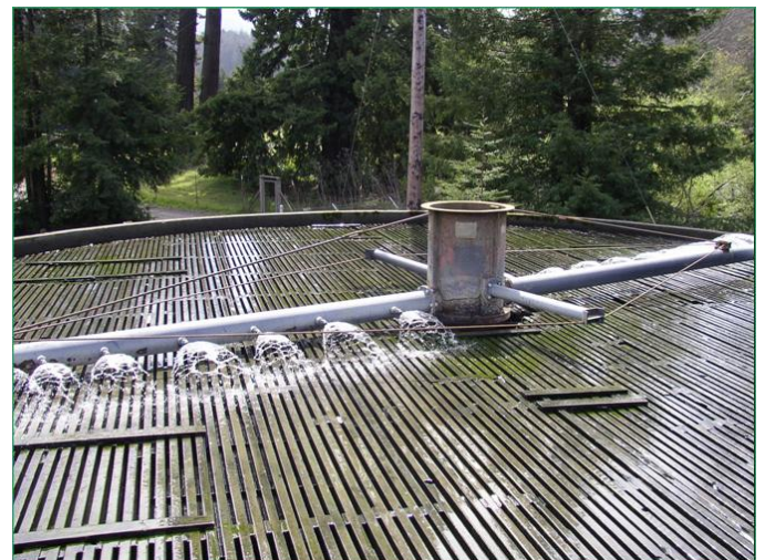
Scotia trickling filter at the wastewater treatment facility.
