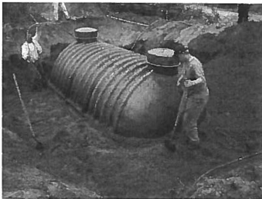
New septic tank at Prairie Creek Redwoods S.P.
