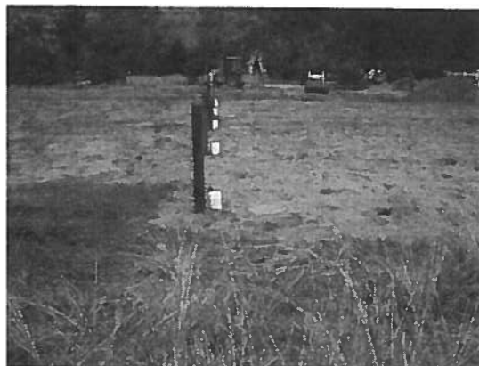
Completed leach field at Prairie Creek.
