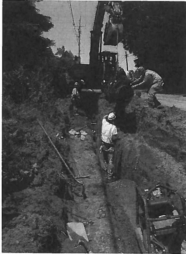
Installation of 18" water main in county road right-of-way.
