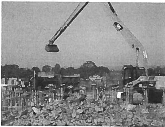
Long reach excavation, backfill and grading.
