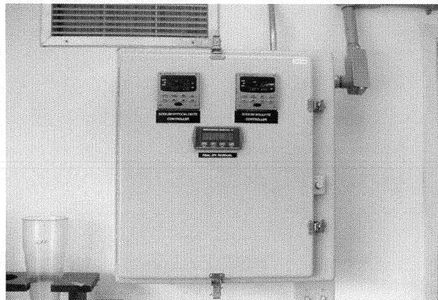
Chlorine Control Panel
